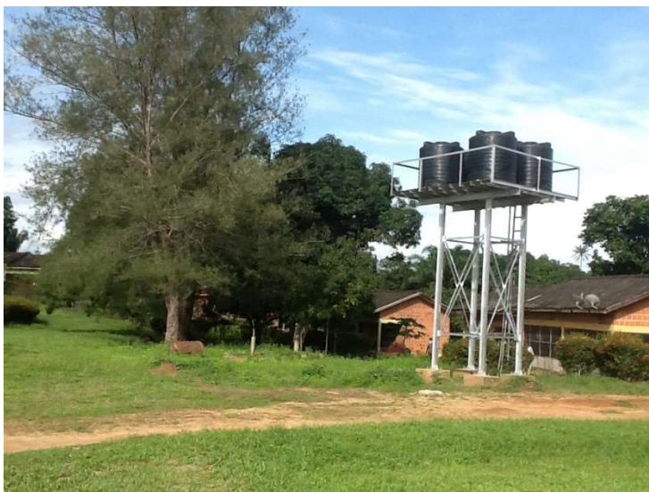
Figure 14: Amaudo water project
